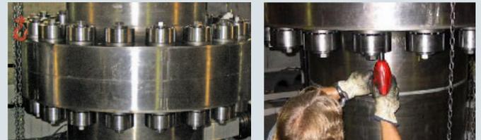
Superbolt Expansion Bolts replaced the tight fitted bolts on this Francis type pump generator shaft coupling at a Hydroelectric pump-storage facility. Compared to the previous conventional bolting method, Superbolt EBs eliminated the unsafe and time consuming installation and removal processes.
